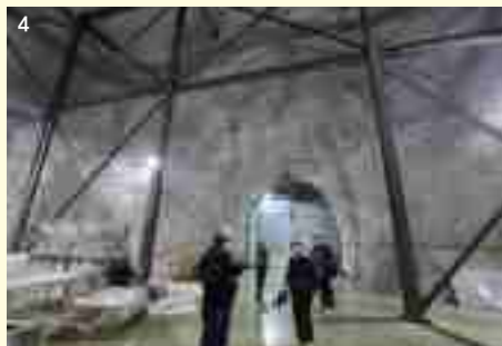
1. Elevator for going down to the underground laboratory. It is 4 times faster than typical apartment elevators. 2. The place that indicates the beginning of YemiLab is marked with a yellow sign for visibility in the dark mine. 3. A neutrino detector will be installed in the LSC cavity, which has a diameter of 20 m and a height of 28 m. 4. The AMoRE experiment team was already installing dust shields and installing equipment while the construction was in the finishing phase. 5. IBS also built a dormitory for researchers after consultation with Jeongseon-gun. 6. The tunnel leading to the underground laboratory is equipped with complex systems for electricity and ventilation. 7. Senior Engineer PARK Kang-Soon provided a guided tour of the YemiLab.
